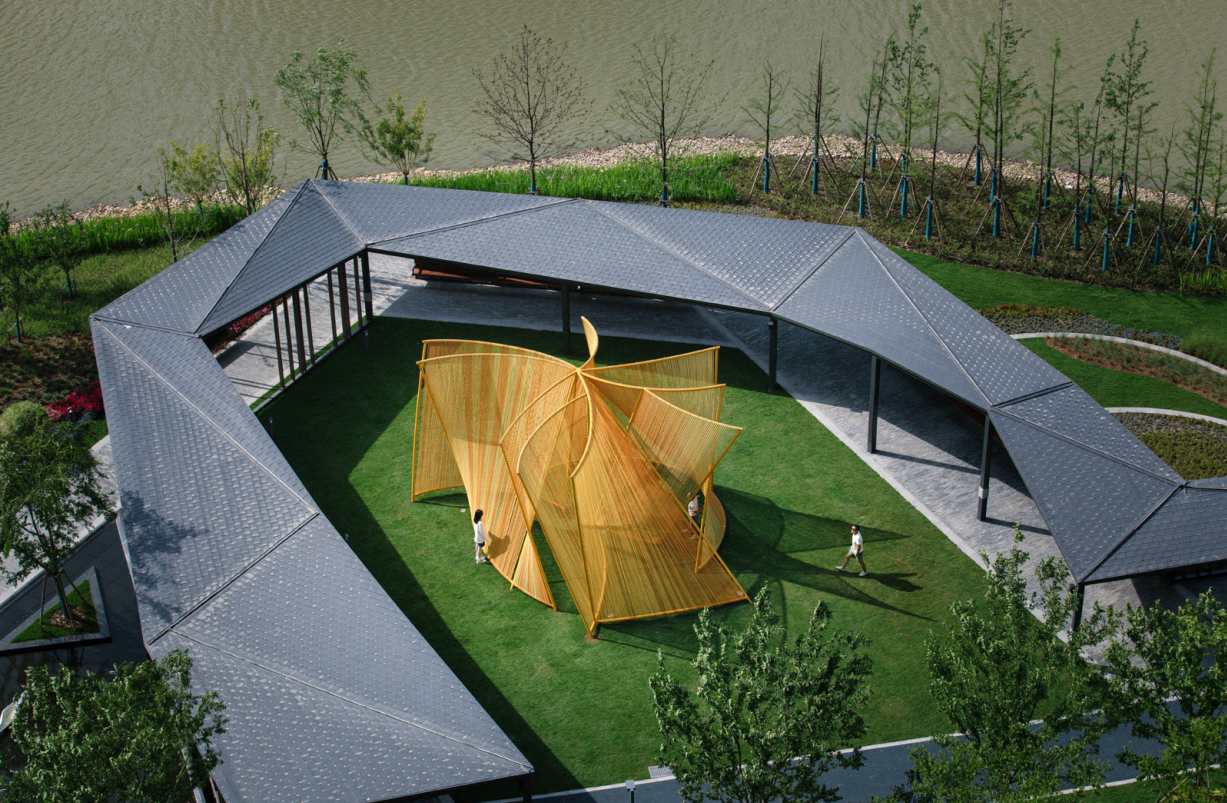
all photos courtesy of Atelier YokYok / credit XiongMan
